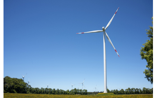
Wind Turbines for power generation
