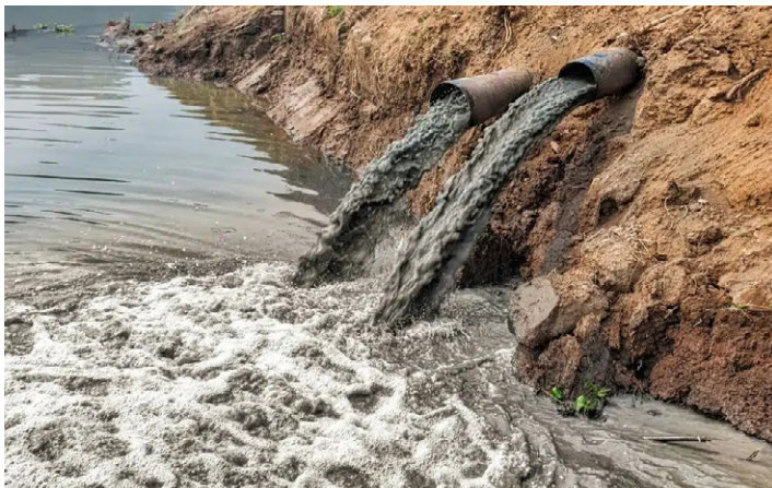
Drains Pouring into the River
