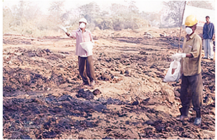
Application of Oilzapper on an oil-spill site in Assam Source: TERI
