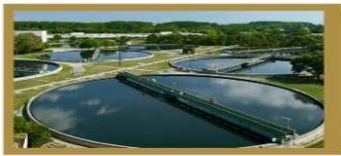
Sewerage Treatment Infrastructure
